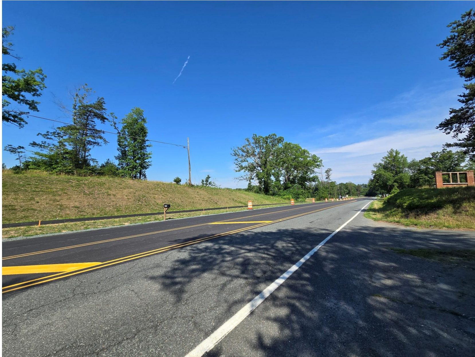
Figure 1d: View looking southwest into the site from the Rt. 250 Entrance Corridor.
